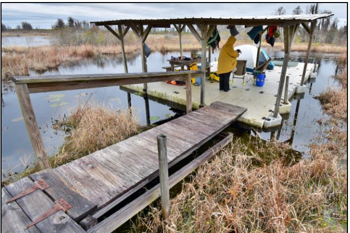
The backside of Cedar Hammock, as seen from where the vault/pit toilet is located.
