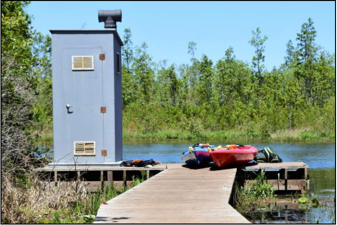
Vault/pit toilet at Monkey Lake. The camping platform is 120 ft. away from this area.
