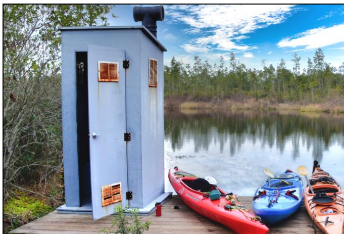
Every campsite and day-use shelter has a vault/pit toilet. Pictured: Monkey Lake camp.
